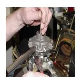
STEP 4 Tighten mounting screw (p/n: 018-1004-93-0) onto valve flange as shown, then tighten stop sleeve (p/n: 159-1990-00-0 onto screw. Installation is complete.
