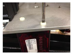
15. Reinsert bolts into panel, and reposition spacers onto bolts.
